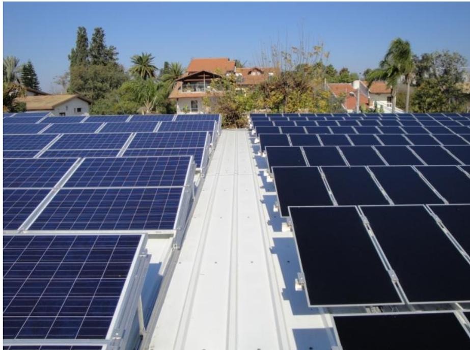
The thin-film technology used is Cadmium Telluride (CdTe), the cSi is a polysilicon product. The same series of inverters are used for both sides of the array, a 9kW for the cSi and an 8kW for the CdTe. The time frame for the study is from July to December, presenting a 6 month cycle indicative of all solar paths over a twelve month period. In order to compare the output as technologically driven, the data was normalized to kWh/kWp/day.
